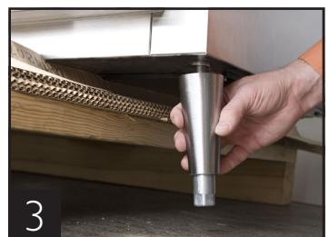
Thread leg into cabinet bottom cabinet.
