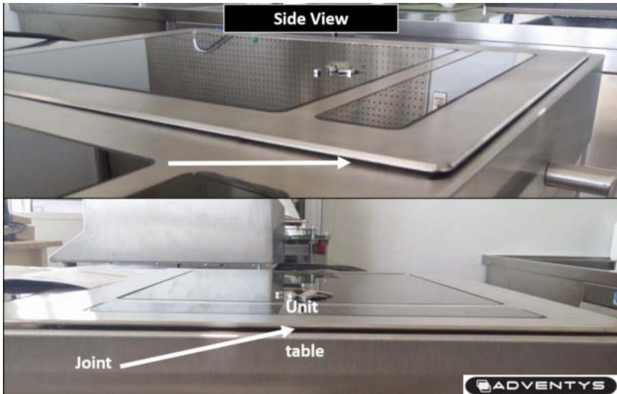
Remove the unit, turn it upside down and place it on a surface which will protect the glass from being scratched. Place a bead of NSF approved high temperature sealant entirely around the outer edge of the underside of the unit to create the joint. Place the unit back into the opening and carefully push into place.
