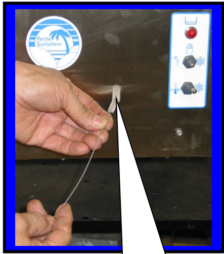
Insert long brush F6526 into drip tube
