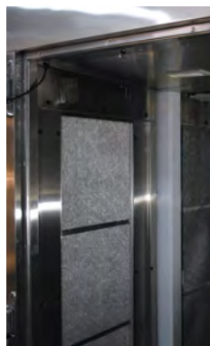
Coil Frame Assembly
