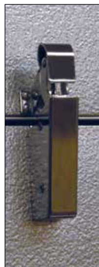
Spring actuated door closer
