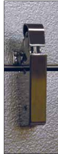
Spring actuated door closer
