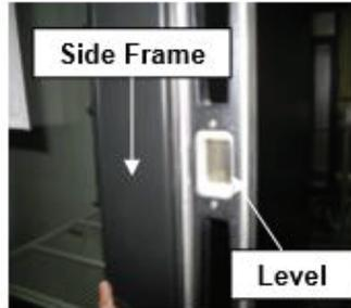
1. To insure proper operation, the cabinet must be level.
